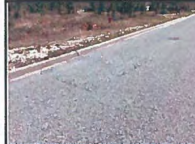
2. Photograph depicting an approximately 8.5 ft. X 7 ft. patch observed in the northbound travel lane near 302 Columbus Street. The pavement transitions were observed to be smooth.
