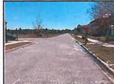
4. Photograph depicting conditions near the intersection with Liverpool Avenue. View to the south.
