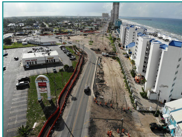
CRA roadway improvements continue along Front Beach Road.
