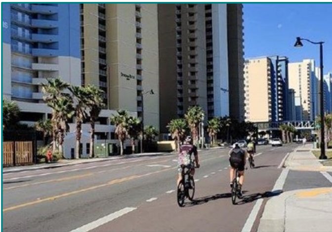
Bicyclists enjoy their own dedicated bicycle lane along completed Segment 2 of the Front Beach Road CRA project.
