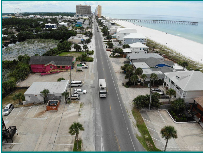
Front Beach Road eastward looking view.
