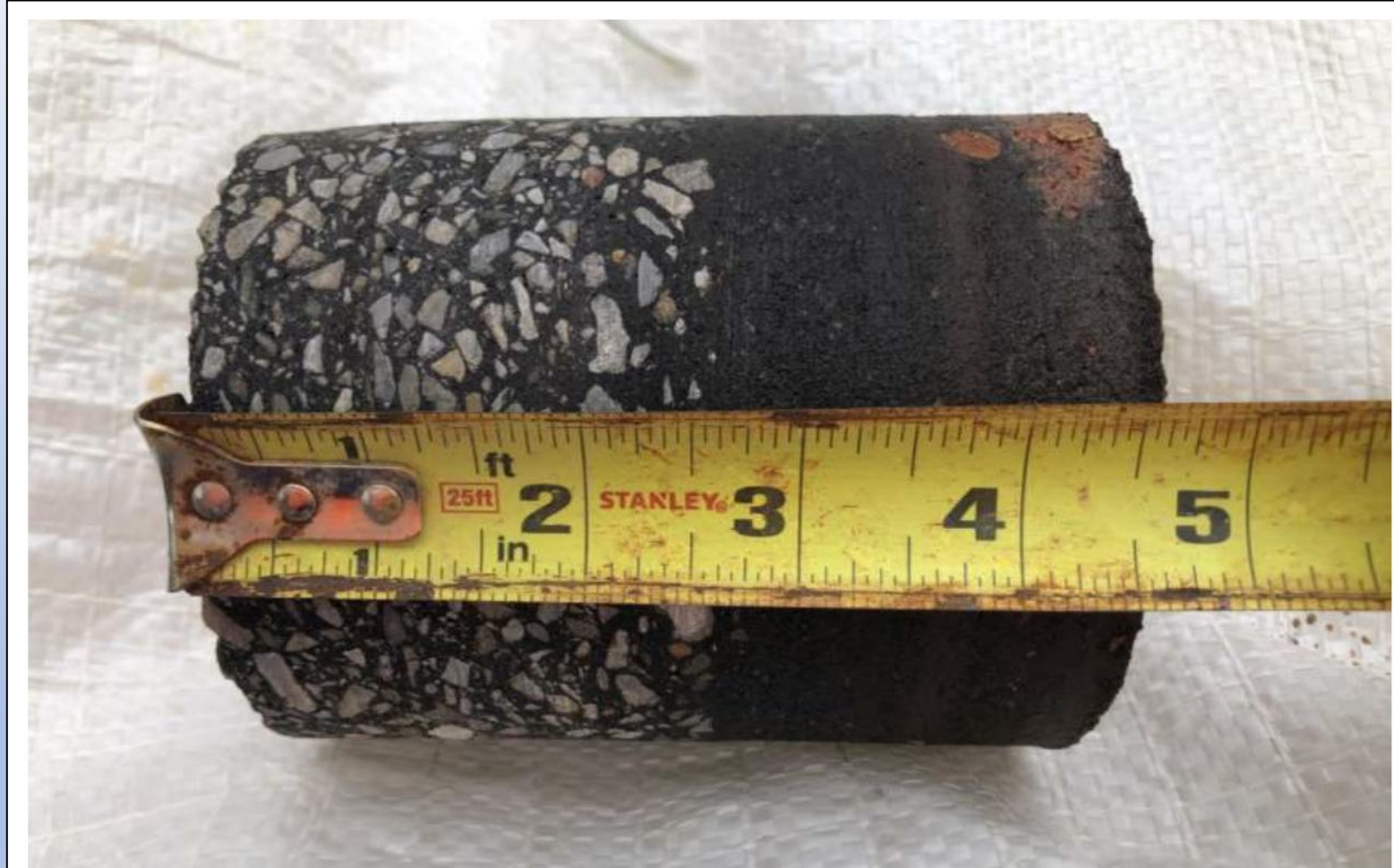
Core C-3 - Approximately 2-5/8 Inches of Asphaltic Concrete and 2 Inches of Sand Asphalt Base
