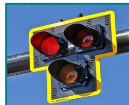
Example of a Pedestrian Hybrid Beacon (PHB)
