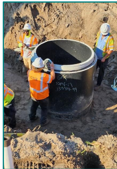
Crews installing a sanitary sewer manhole riser section at Guava Ave.
