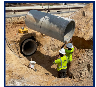
Contractor crew undergrounding utilities July 28, 2023.
