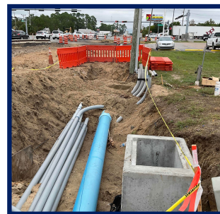
Contractor is performing open site excavation in order to install a new water main on South Arnold Road.
