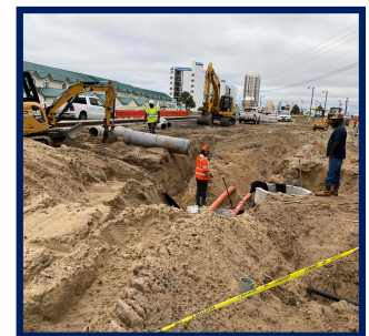
Contractor is performing open site excavation in order to install a new water main on South Arnold Road.
