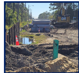
Glimpse of work on the road closure area so far.
