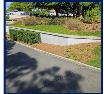
Typical retaining walls
