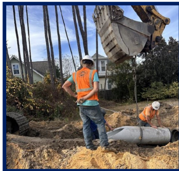
Installing the RCP pipe.
