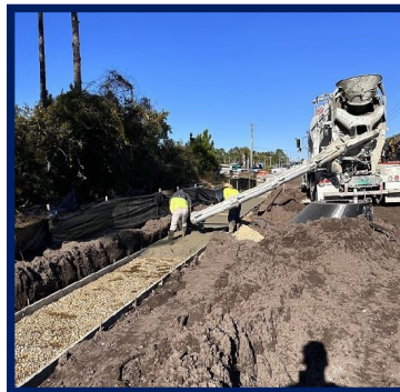
Placing concrete for the gravity wall.
