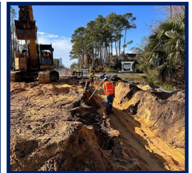
Backfilling materials around the RCP pipe.
