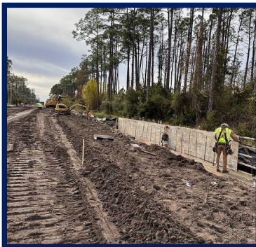
Constructing footings for the gravity wall.
