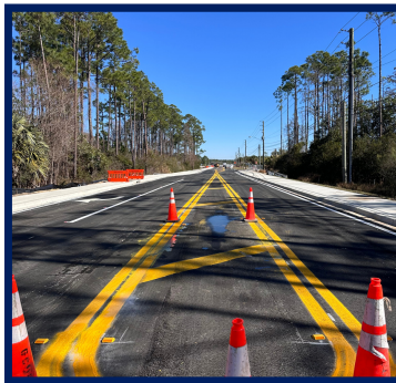
Road raised ~18 inches, improved drainage, upgraded sidewalks and fresh pavement/stripping.
