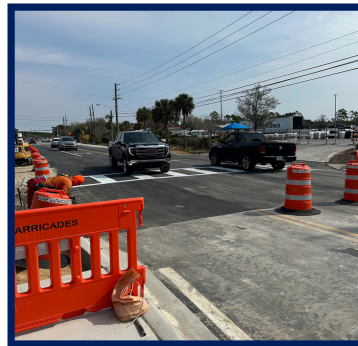
Road raised ~18 inches, improved drainage, upgraded sidewalks and fresh pavement/stripping.
