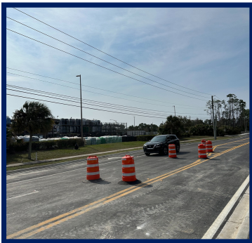
Road raised ~18 inches, improved drainage, upgraded sidewalks and fresh pavement/stripping.
