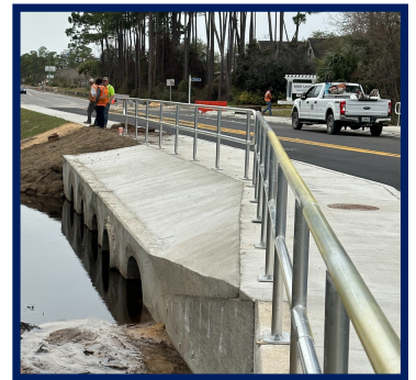
Upgraded culverts and sidewalks just north of Cabana Boulevard.
