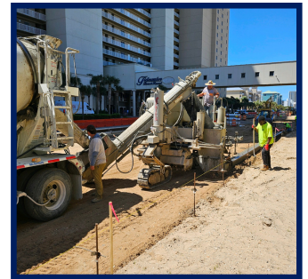
Placing curb in the area of Tidewater Beach Resorts.
