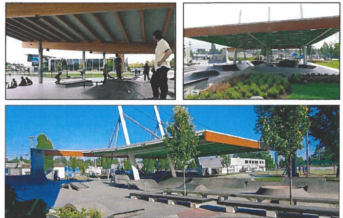
Covered structures from our Cloverdale and Chuck Bailey covered youth park projects
