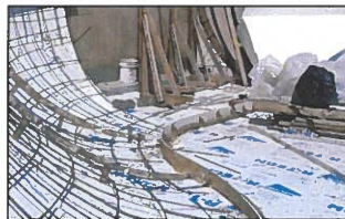
Light-Weight Structural Styrofoam Sub Base Queensborough All-Wheel Park - New Westminster, BC and Seattle Center Skate Plaza - Seattle, WA
