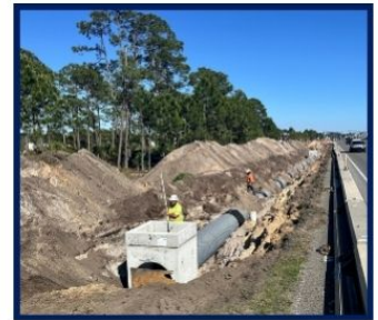
New drainage pipes being installed along U.S. 98.
