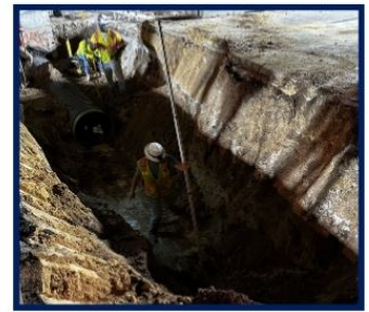
New drainage pipes being installed along U.S. 98.
