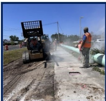
Removing damaged sidewalk, building forms to place the new sidewalk, and placing concrete for new curbing in the CVS area.
