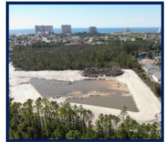
Retention pond taking shape behind Harley-Davidson.
