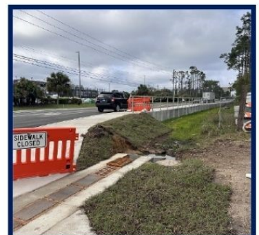
Placing sod along the new trench drain at the Dairy Queen driveway.
