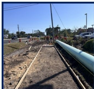
Removing damaged sidewalk, building forms to place the new sidewalk, and placing concrete for new curbing in the CVS area.
