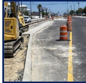
Median work north of the roundabout.
