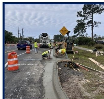
Removing damaged sidewalk, building forms to place the new sidewalk, and placing concrete for new curbing in the CVS area.
