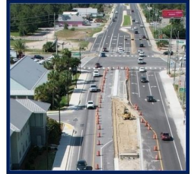
A median correction to its approved elevation is ongoing at the intersection of S. Arnold Road and U.S. 98. This reconstruction is at no cost to the City.
