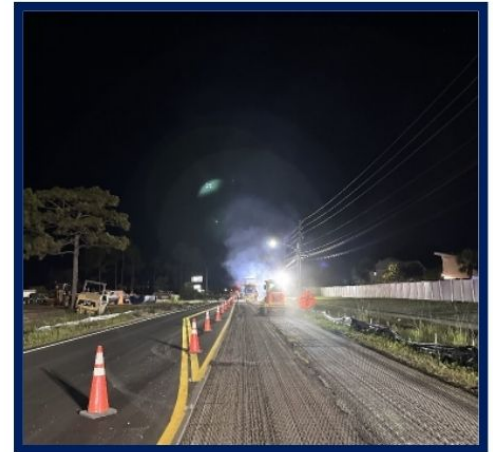
Milling asphalt near Moonraker Circle.
