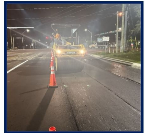
Compacting new asphalt near the intersection with Hutchison Boulevard.
