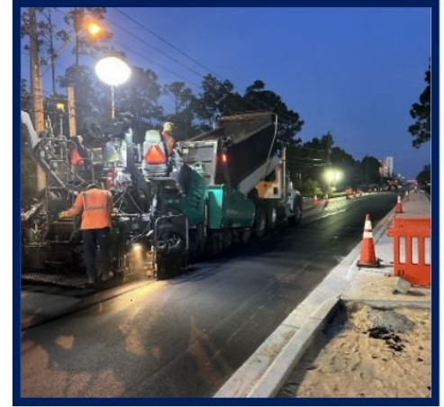
Paving the median turn lane near Cabana Boulevard.
