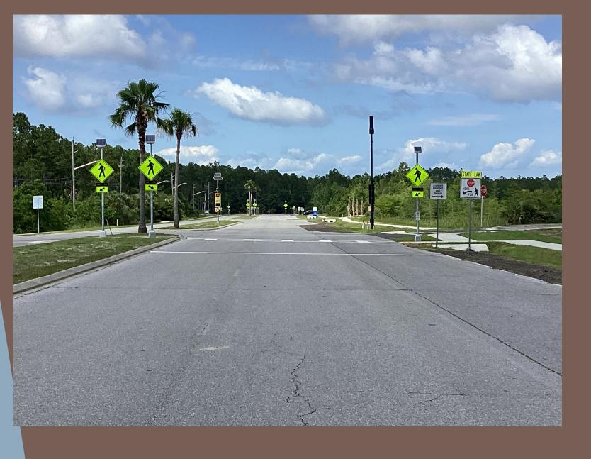
Crosswalks RRFB's and associated striping were installed using City staff to complete this project
