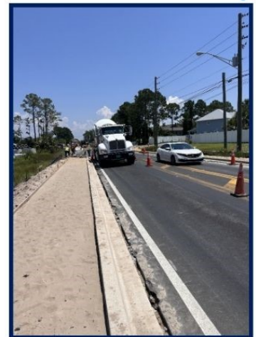
Constructing new curbing and sidewalk in the area of the Church of Christ and across from Moonraker Circle.
