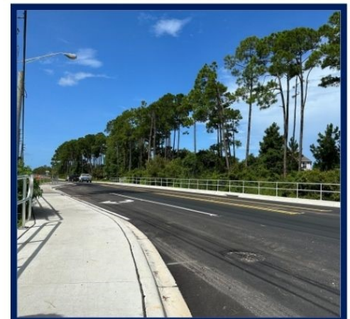
Handrails where needed and wider, continuous sidewalks.
