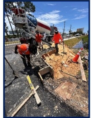
Constructing new curbing and sidewalk in the area of the Church of Christ and across from Moonraker Circle.
