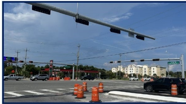
South Arnold Road/U.S. 98 intersection.
