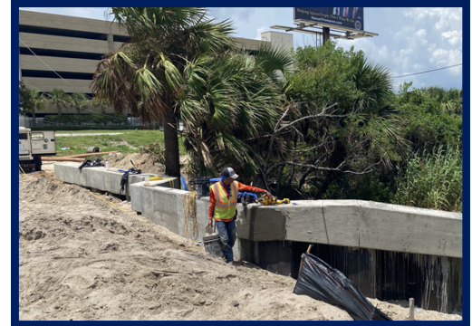
Lullwater Lake weir construction.
